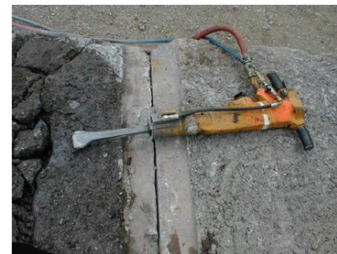
Jackhammer equipped with water spray delivery system to control dust. The water nozzle is mounted on the jackhammer frame just to the right of the chisel. Note the wet concrete on left from the water spray.
