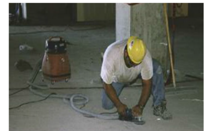
Worker grinding concrete floor with grinder attached to dust collector (background).
